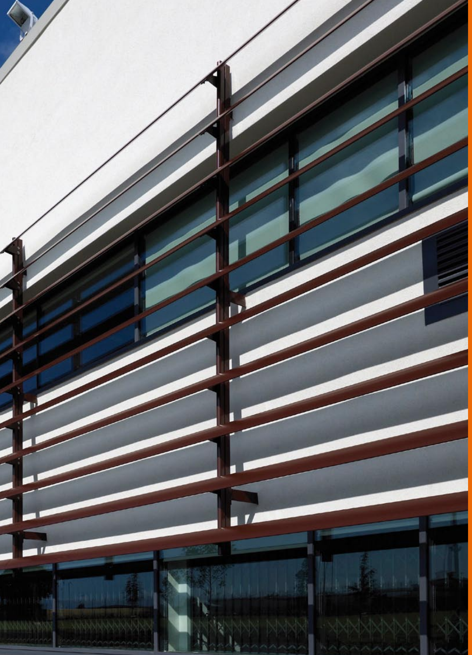
Above: South Sefton Sixth Form College finished with Hanson Structherm's Thin Coat System
